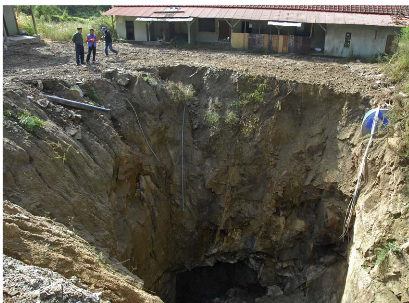
Fig. 2. The open collapse hole over the old Mookkeuk gold mine, looking south along the line of the vein, in late 2009.
