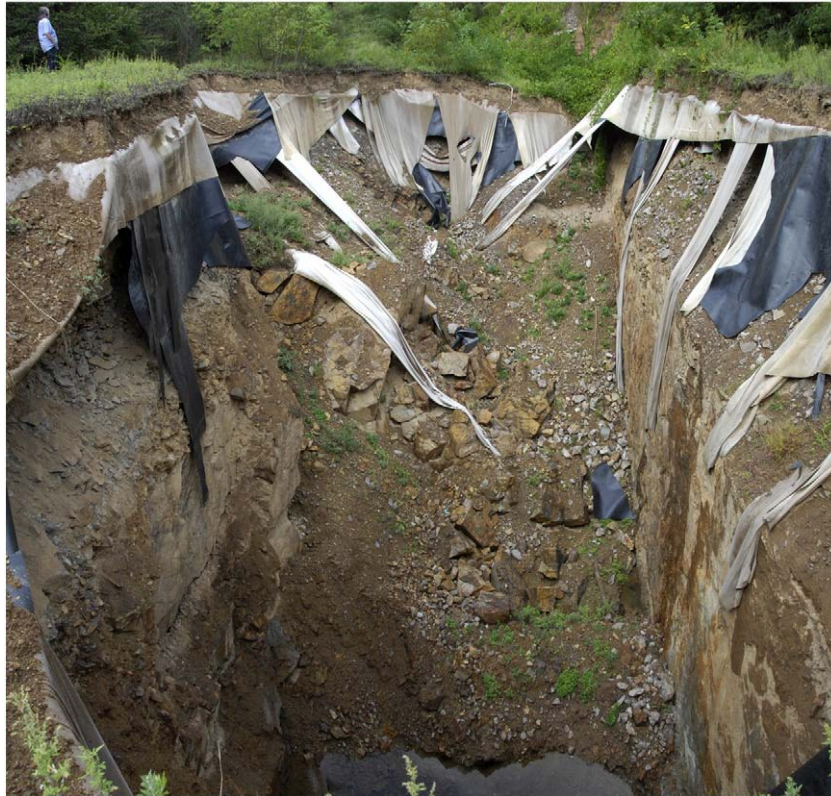
Fig. 8. The collapse sinkhole at the old Toehyun mine, looking north, after it was enlarged during the 2009 earthquake. Broken strips of geotextile, placed beneath the soil during site reclamation, hang down the walls.
