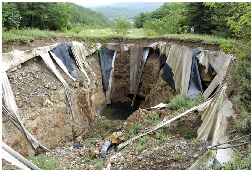
Fig. 9. The large collapse sinkhole at the old Toehyun mine, looking south, down the valley, after the earthquake.
